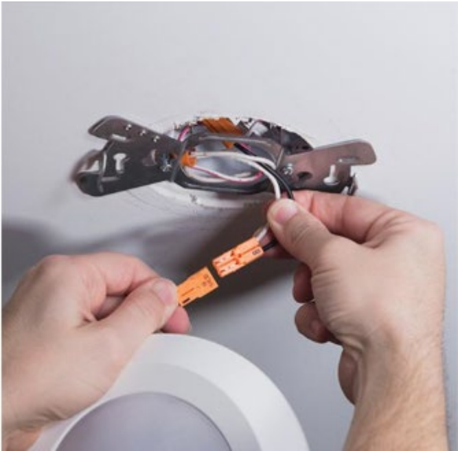
LED surface mounted light fixture with an air sealed electrical box:
