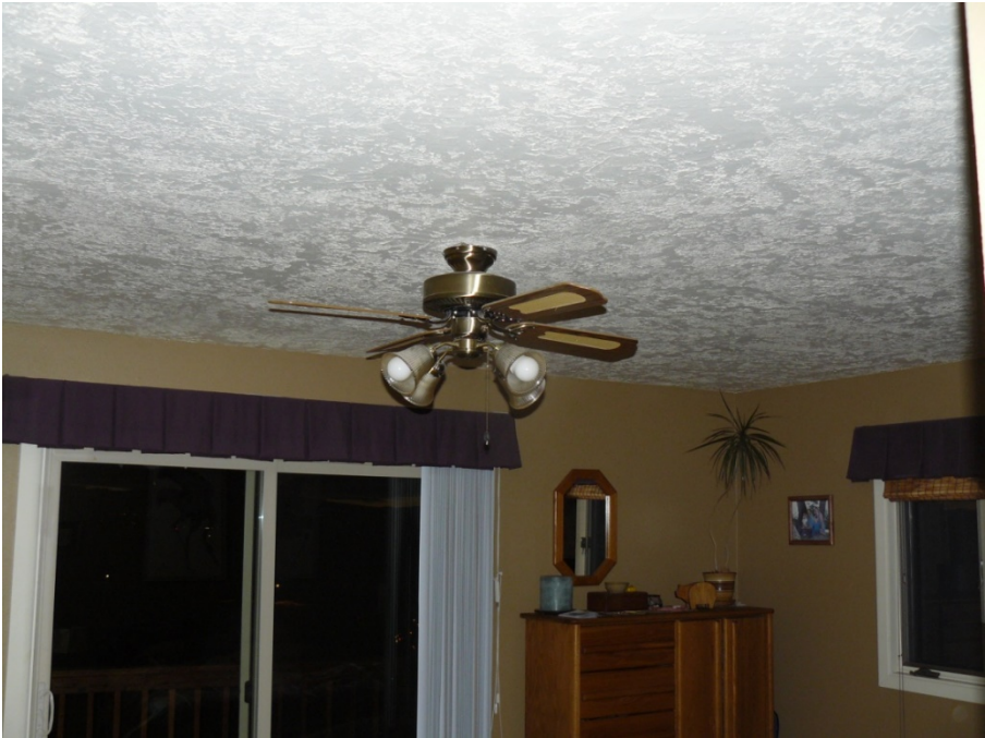
Air leakage at ceiling fan:
