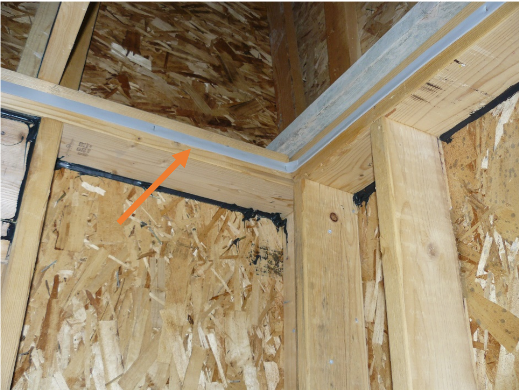
Fix: top plate gasket sealing gap between sheetrock and top plate:
