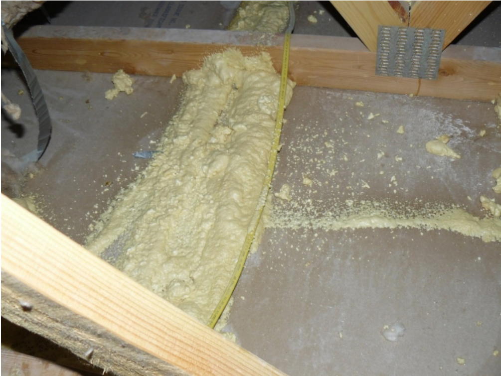
Fix: top plate gasket sealing gap between sheetrock and top plate:
