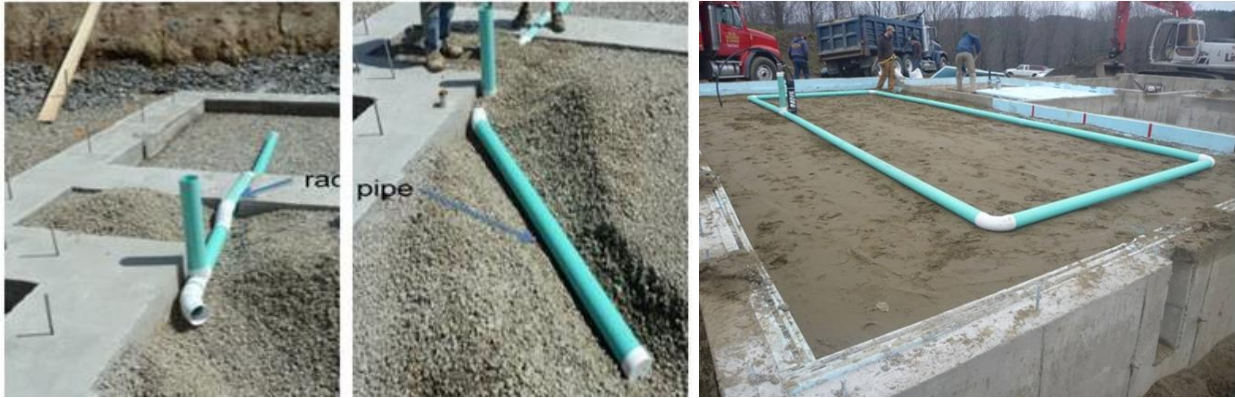
Perforated Pipe Being Installed Below Slab
