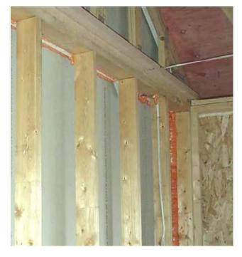
Example of properly air sealed common wall with fire-rated sealant (in orange). Source: ENERGY STAR Thermal Bypass Checklist Guide and MaGrann Associates
