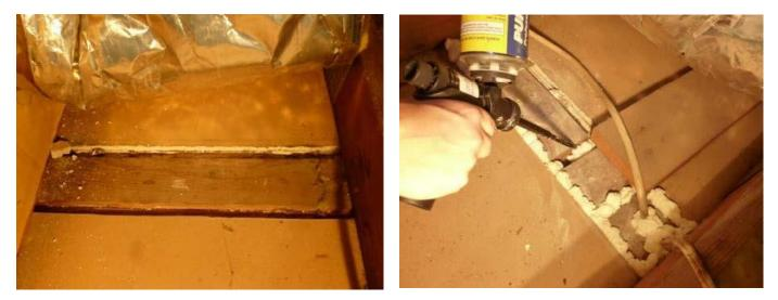
In the photo on the left, gaps on each side of a common wall are left unsealed. On the right, fire rated spray foam is used to seal those gaps at the top plates.
