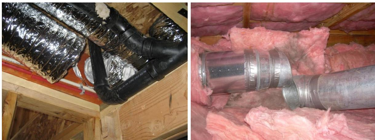
Duct tightness testing will identify significant duct problems such as disconnected duct joints. This is one reason why duct tightness testing is good practice even when all of the ducts are located within the building thermal envelope.
