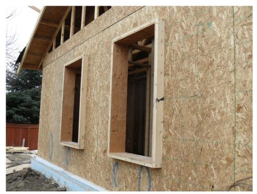
Exterior walls have R-21 fiberglass batt in the wall cavity and two layers of R-10 foam sheathing with seams taped on each layer for total wall of R-41.
