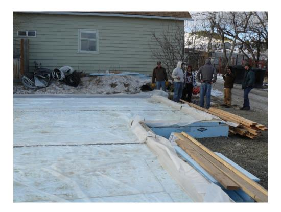
2 feet horizontal layer of R-10 prevents frost from getting under the foundation.
