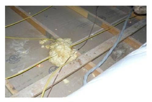
Montana DEQ conducted several trainings at the house with a blower door and infrared camera. Here Youth Build students detect slight air leakage at an exterior wall electrical outlet.
