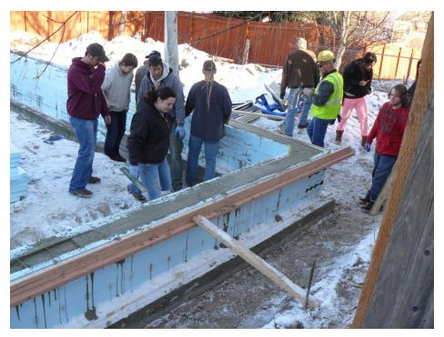
2 layers of 2-inch DOW board (insulating value of R-20) was placed under the entire under floor.
