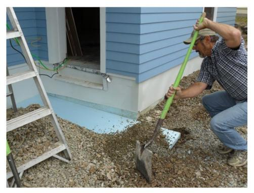
Wall extension framing for windows, ready for 4 inches of DOW board (R-20) foam sheathing.
