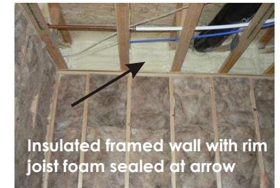
Insulated framed wall with rim joist foam sealed at arrow
