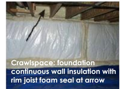
Crawlspace: foundation continuous wall insulation with rim joist foam seal at arrow
