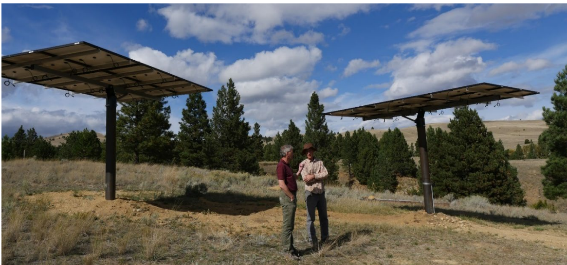
DEQ staff visit FY19-funded off-grid array under construction outside Helena
