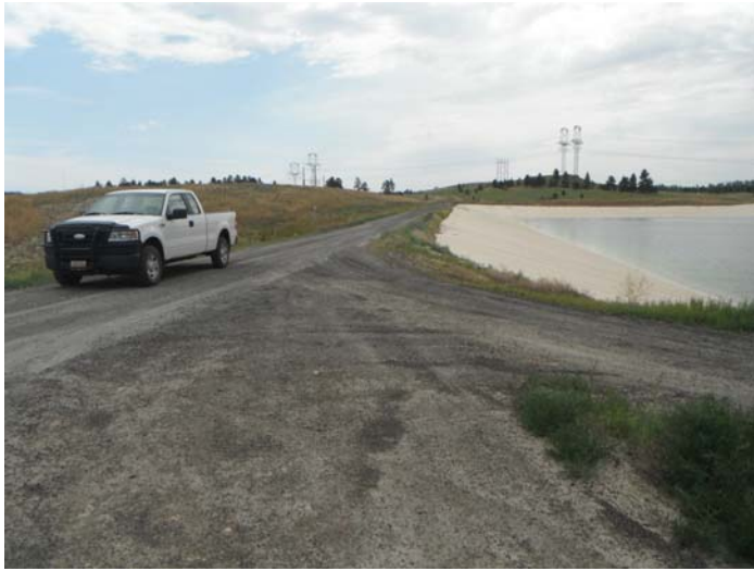
Photo 1. Units 1 & 2 STEP Main Dam, July 15, 2014. New Cell D liner and fill on downstream side of dam.
