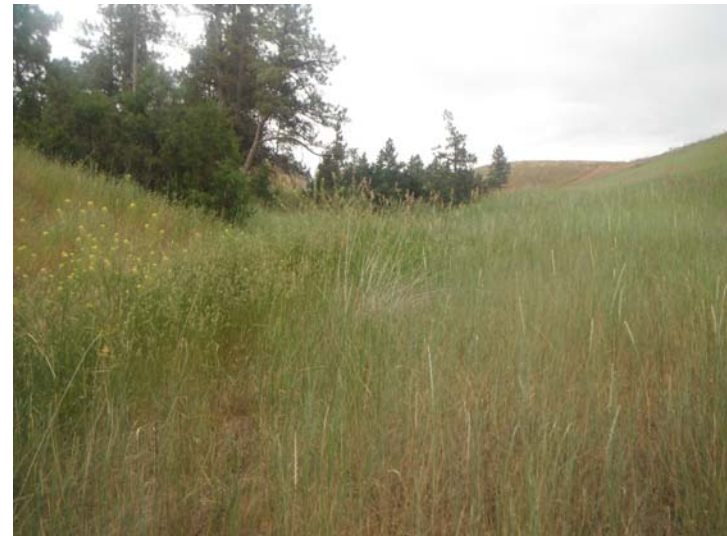
Photo 16. Units 1 & 2 STEP Main Dam, July 15, 2014. Downstream toe, right groin area, erosion repaired.
