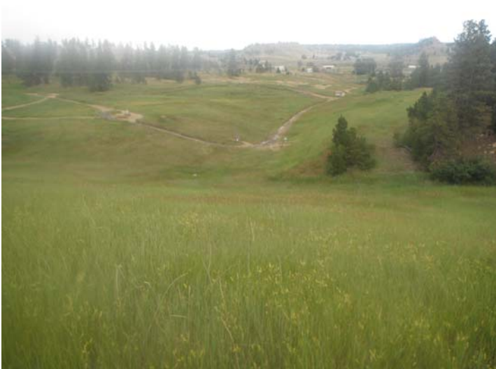
Photo 7. Units 1 & 2 STEP Main Dam, July 15, 2014. Downstream slope and toe area.
