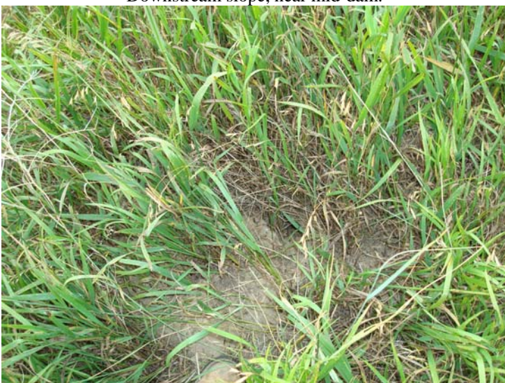
Photo 27. Units 1 & 2 STEP Main Dam, July 15, 2014. Rodent hole, downstream slope.
