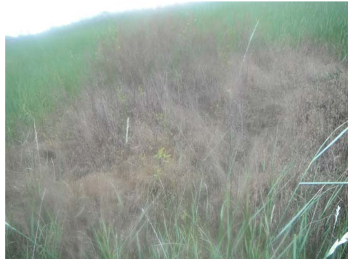
Photo 4. Units 1 & 2 STEP Main Dam, July 15, 2014. Downstream slope, dry, weedy patch typical around rodent holes.
