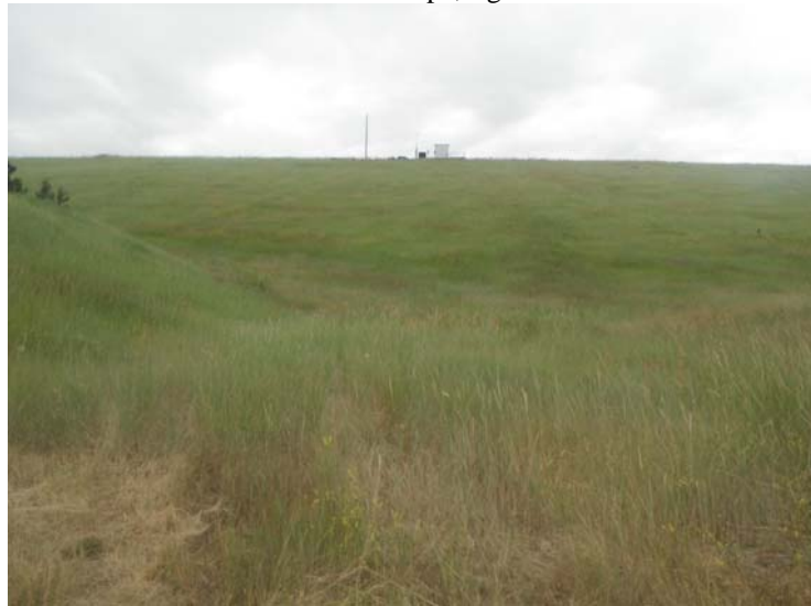
Photo 23. Units 1 & 2 STEP Main Dam, July 15, 2014. Downstream slope.
