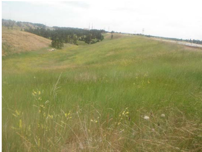
Photo 11. Units 1 & 2 STEP Main Dam, July 15, 2014. Downstream slope from left abutment.
