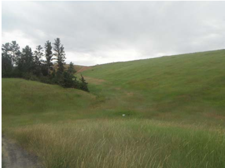
Photo 21. Units 1 & 2 STEP Main Dam, July 15, 2014. Downstream slope, right side.
