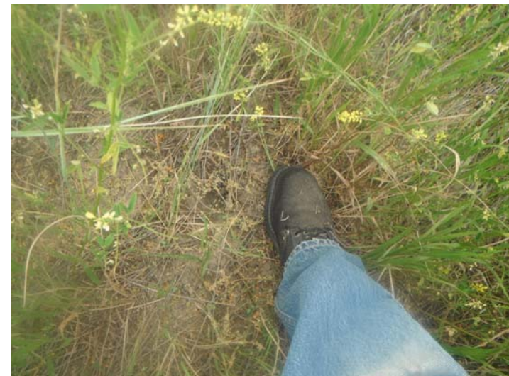
Photo 8. Units 1 & 2 STEP Main Dam, July 15, 2014. Rodent hole, downstream slope.
