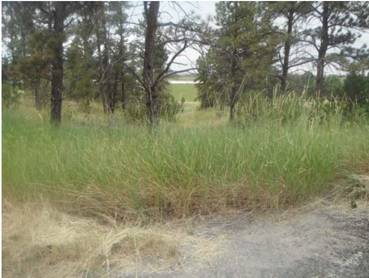
Photo 13. Units 1 & 2 STEP Main Dam, July 15, 2014. Spillway, looking upstream.
