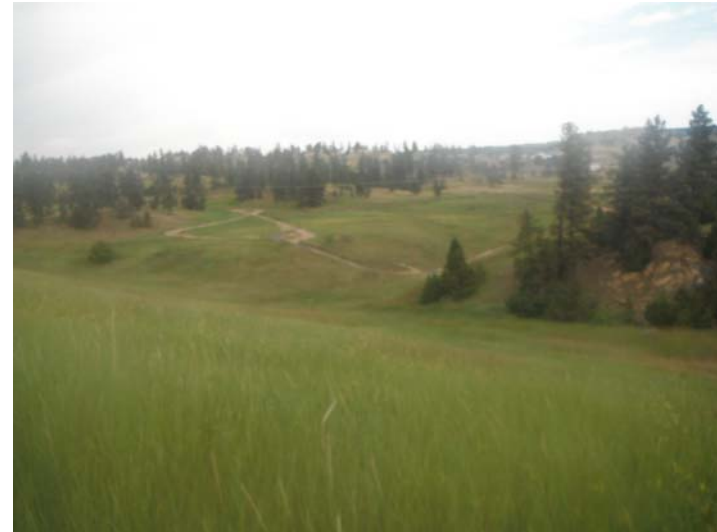
Photo 6. Units 1 & 2 STEP Main Dam, July 15, 2014. Downstream slope and toe area.
