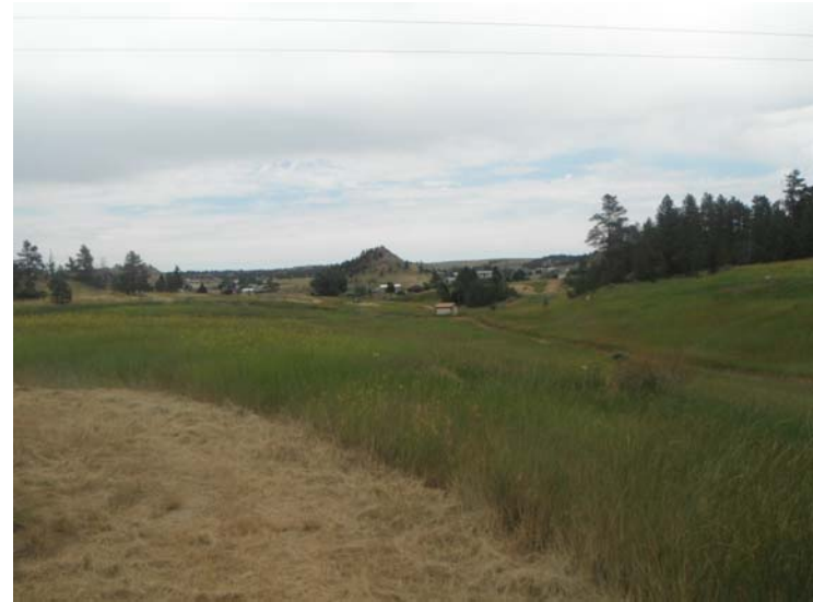
Photo 22. Units 1 & 2 STEP Main Dam, July 15, 2014. Downstream area.
