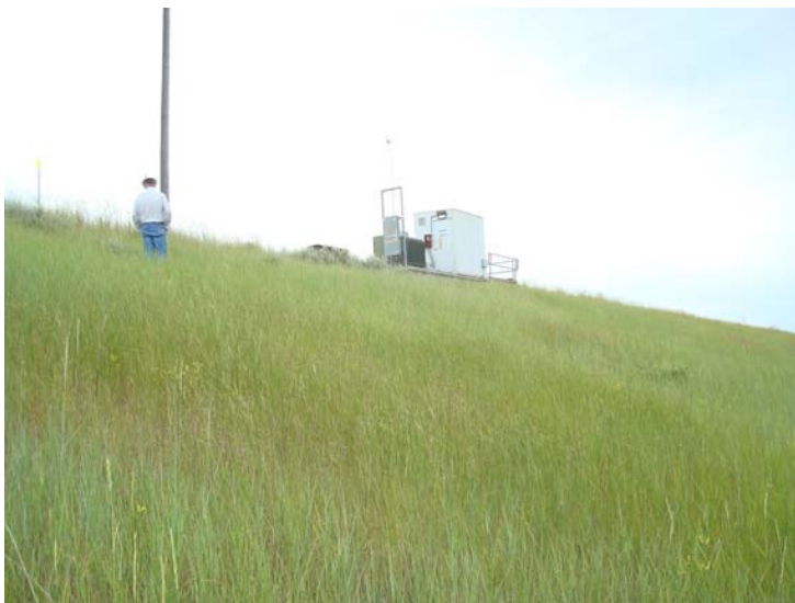
Photo 25. Units 1 & 2 STEP Main Dam, July 15, 2014. Downstream slope, near mid-dam.
