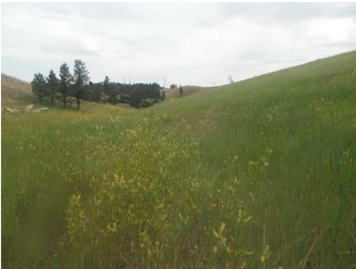
Photo 15. Units 1 & 2 STEP Main Dam, July 15, 2014. Downstream slope and right abutment.
