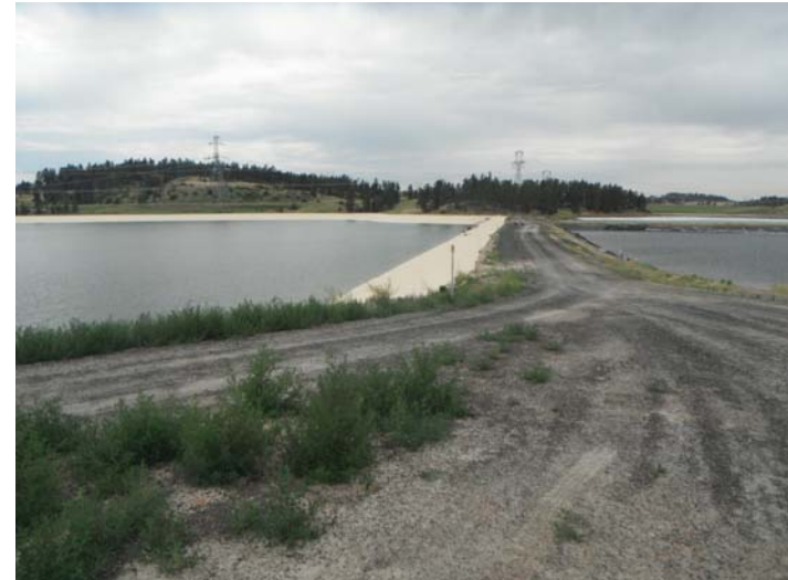
Photo 2. Units 1 & 2 STEP Main Dam, July 15, 2014. New Cell D liner on north side.
