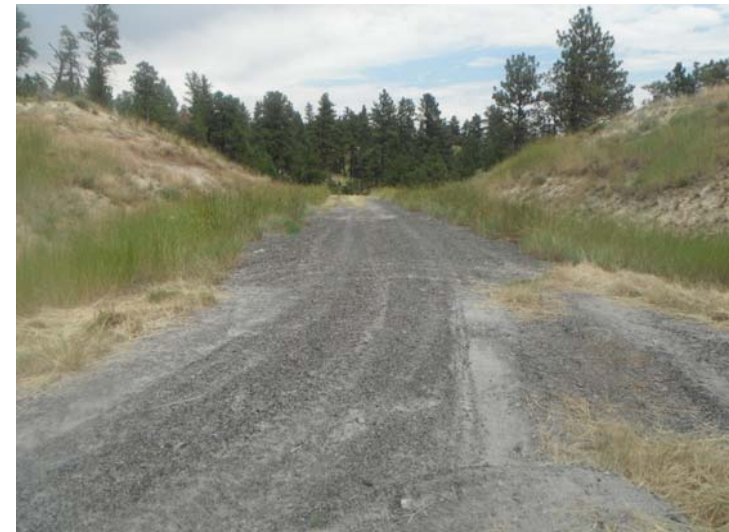
Photo 12. Units 1 & 2 STEP Main Dam, July 15, 2014. Spillway, looking downstream.
