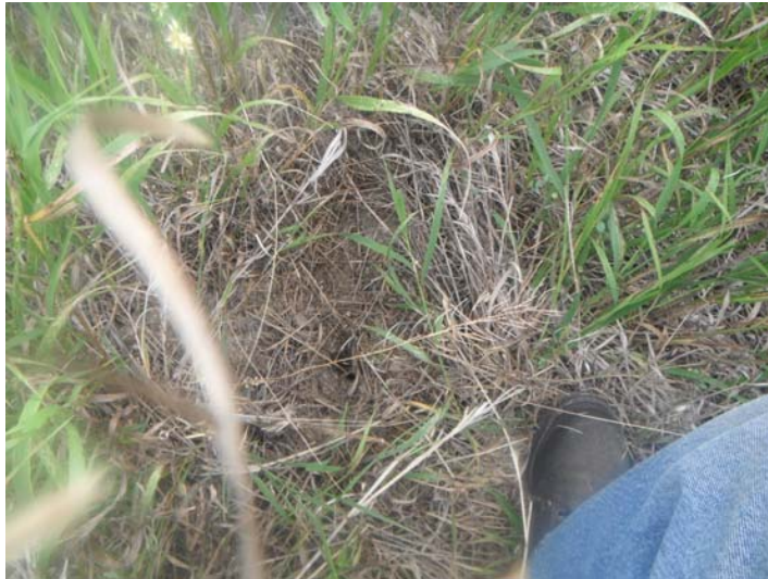
Photo 9. Units 1 & 2 STEP Main Dam, July 15, 2014. Rodent hole, downstream slope.
