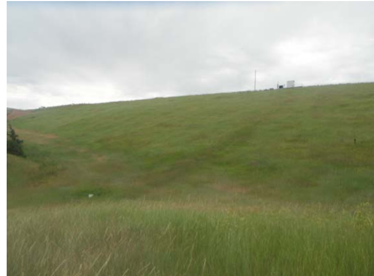
Photo 20. Units 1 & 2 STEP Main Dam, July 15, 2014. Downstream slope, mid-right side.
