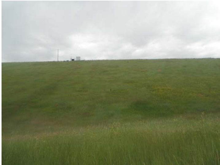
Photo 19. Units 1 & 2 STEP Main Dam, July 15, 2014. Downstream slope, mid-left side.
