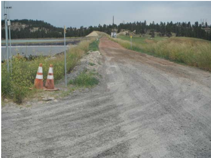
Photo 3. Units 1 & 2 STEP Main Dam, July 15, 2014. Crest from right abutment.
