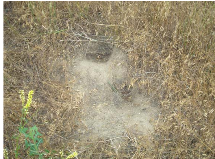
Photo 24. Units 1 & 2 STEP Main Dam, July 15, 2014. Rodent hole, dead grass on downstream slope.
