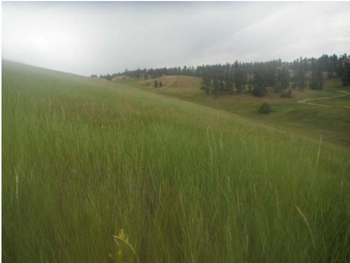
Photo 5. Units 1 & 2 STEP Main Dam, July 15, 2014. Downstream slope from right side.
