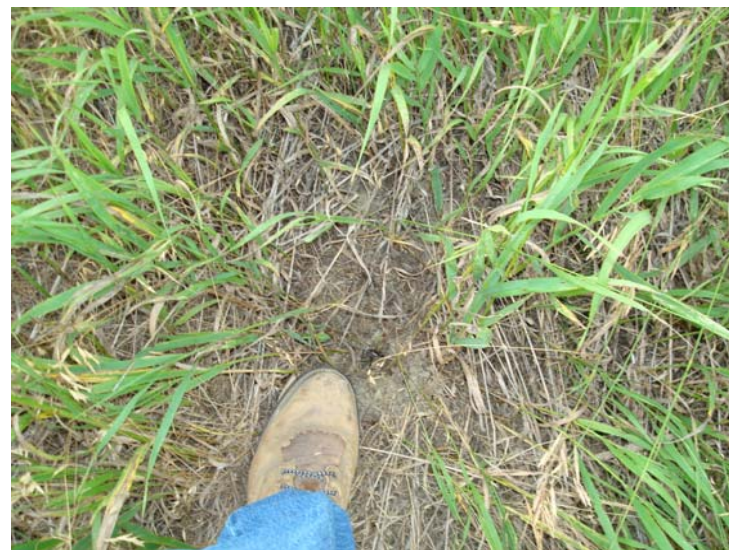
Photo 26. Units 1 & 2 STEP Main Dam, July 15, 2014. Rodent hole, downstream slope.
