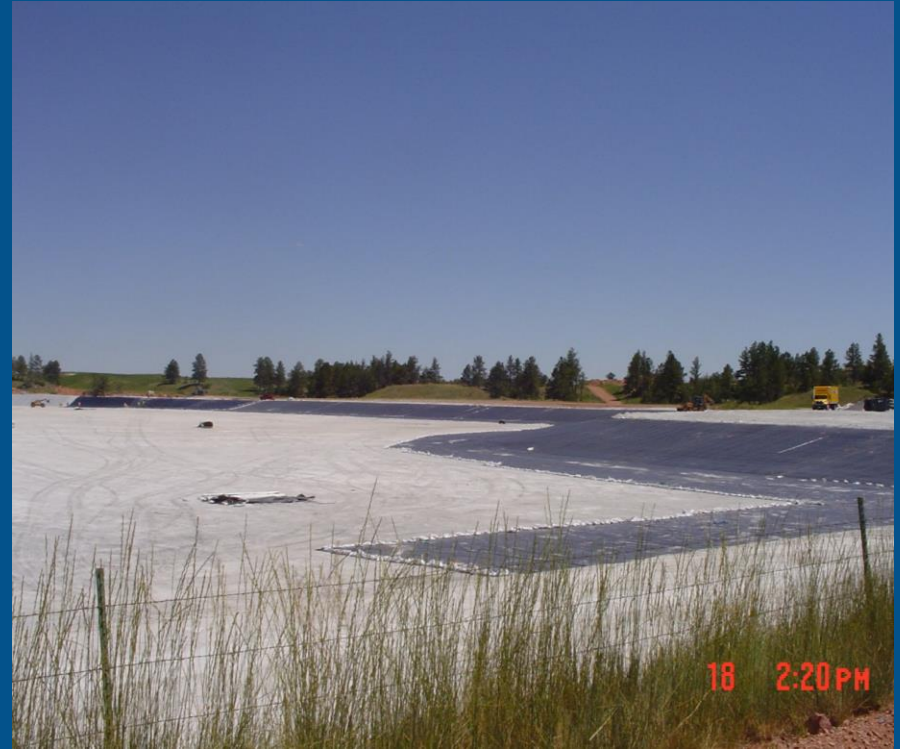
Lining F Cell, Units 3&4 Area, 2005
