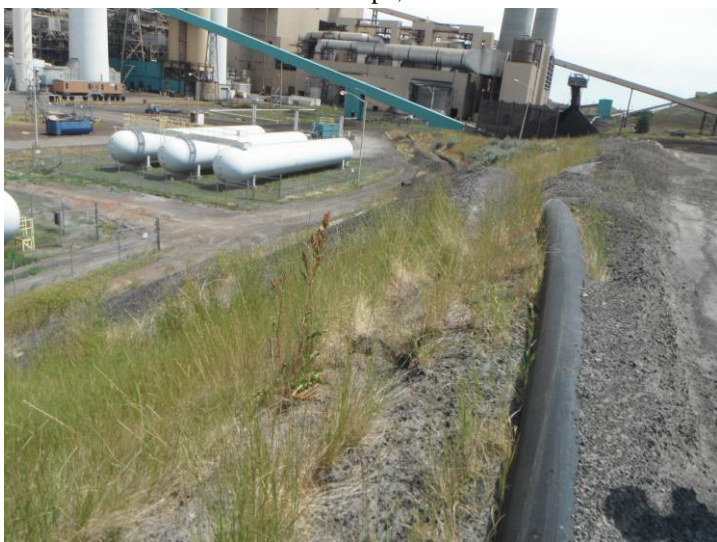
Photo 43. Pond AB Dike, July 15, 2014. Old seepage area, repaired, north dike.
