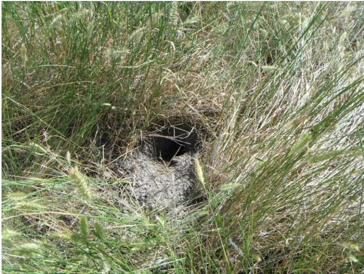
Photo 13. Pond AB Dike, July 15, 2014. Downstream slope, south side of west dike, rodent hole.
