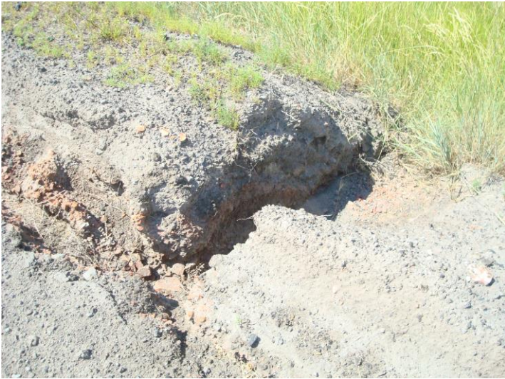
Photo 9. Pond AB Dike, July 15, 2014. Erosion on downstream shoulder of crest, west dike.
