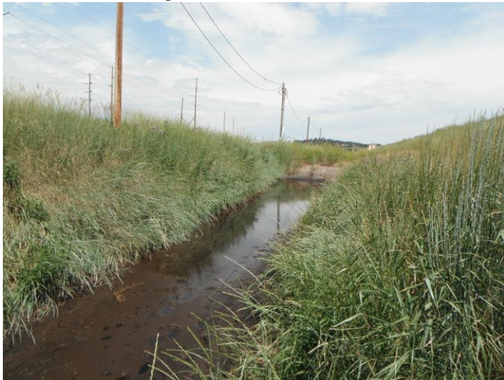
Photo 15. Pond AB Dike, July 15, 2014. Downstream slope, south side of west dike, seepage or runoff ponded.
