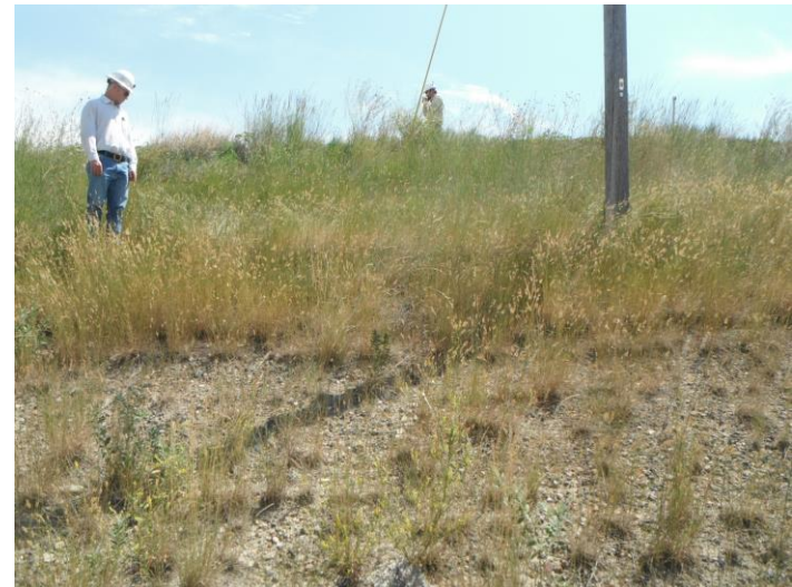
Photo 12. Pond AB Dike, July 15, 2014. Downstream slope, south side of west dike, rodent holes by person.
