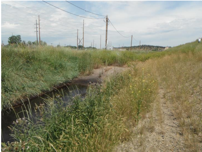
Photo 17. Pond AB Dike, July 15, 2014. Downstream slope, south side of west embankment, seepage/runoff ponding.
