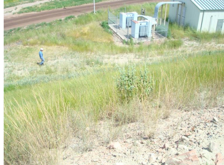
Photo 34. Pond AB Dike, July 15, 2014. Downstream slope, northwest corner, woody vegetation near crest.
