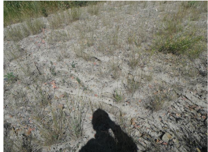
Photo 14. Pond AB Dike, July 15, 2014. Downstream slope, south side of west dike, erosion rills near toe.
