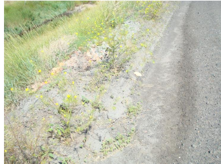
Photo 6. Pond AB Dike, July 15, 2014. Erosion on downstream shoulder of crest, west dike.
