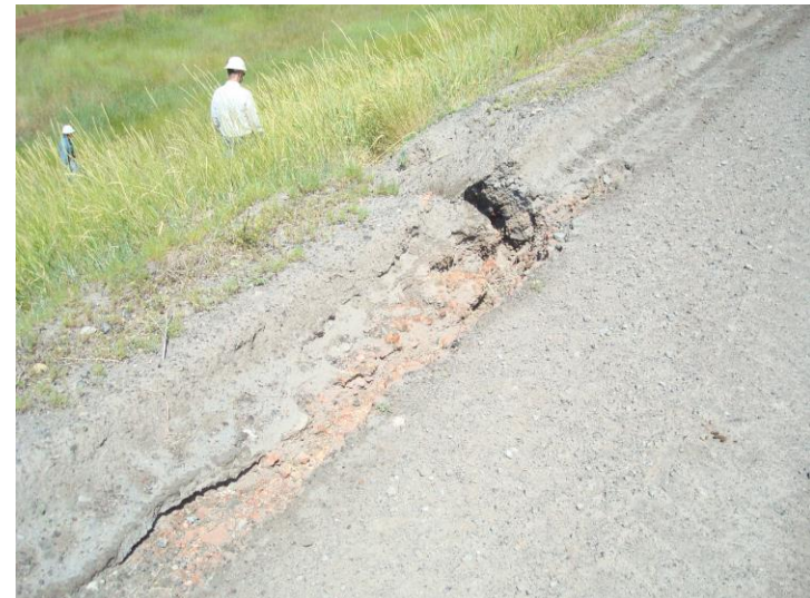
Photo 8. Pond AB Dike, July 15, 2014. Erosion on downstream shoulder of crest, west dike.
