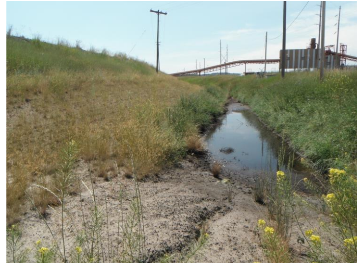
Photo 18. Pond AB Dike, July 15, 2014. Downstream slope, south side of west embankment, seepage/runoff ponding.
