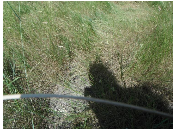
Photo 20. Pond AB Dike, July 15, 2014. Rodent hole, downstream toe, middle of west dike.
