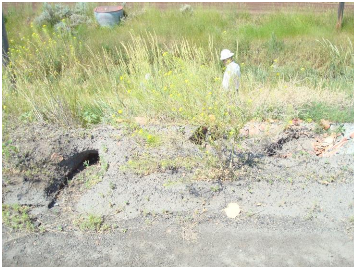
Photo 7. Pond AB Dike, July 15, 2014. Erosion on downstream shoulder of crest, west dike.
