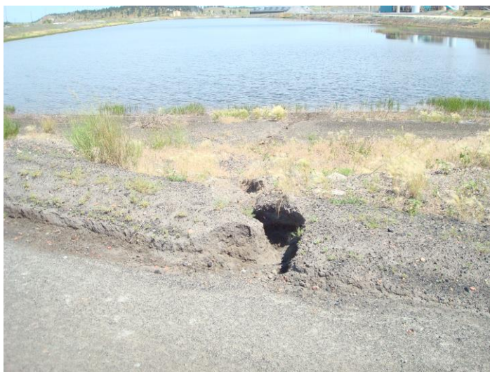
Photo 1. Pond AB Dike, July 15, 2014. Crest, south dike, erosion on inboard shoulder.
