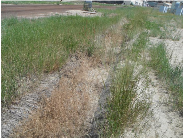
Photo 31. Pond AB Dike, July 15, 2014. Drainage channel in downstream toe, northwest corner.
