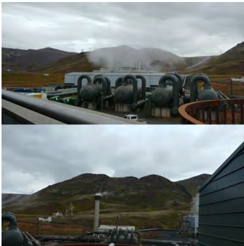
Hellsheiði Geothermal Power Station sits atop basalt-rich formations. Credit: Kimberly M. S.
