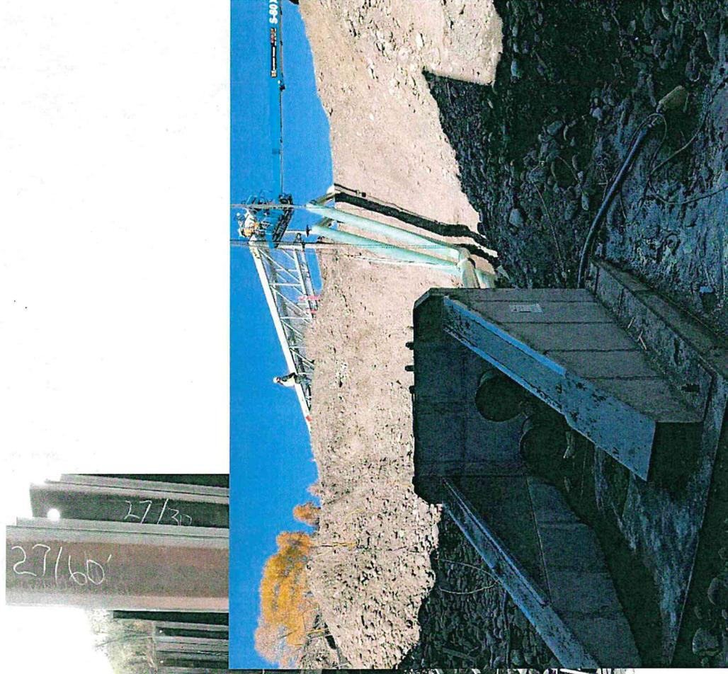
Sheet pile and multiple pumps used to allow the diffuser to be safely and securely installed on the river bottom.
