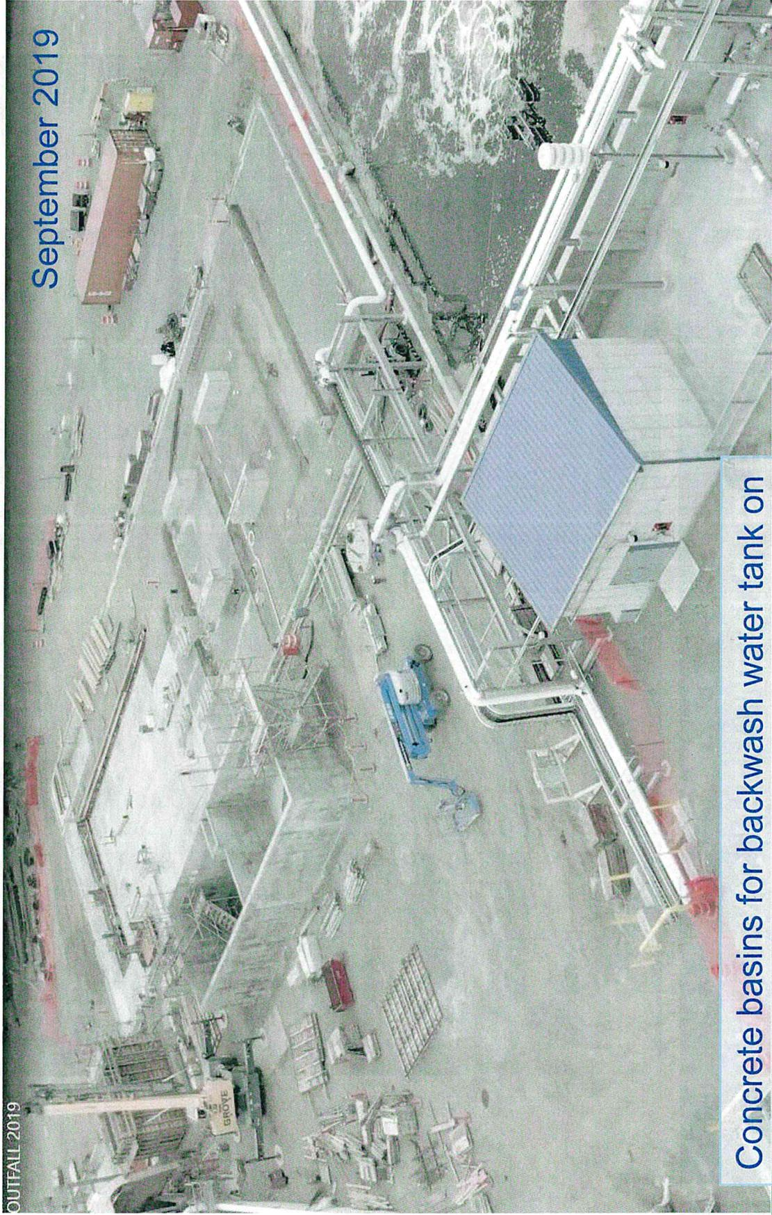
Concrete basins for backwash water tank on the left and supports for filter vessels right.
