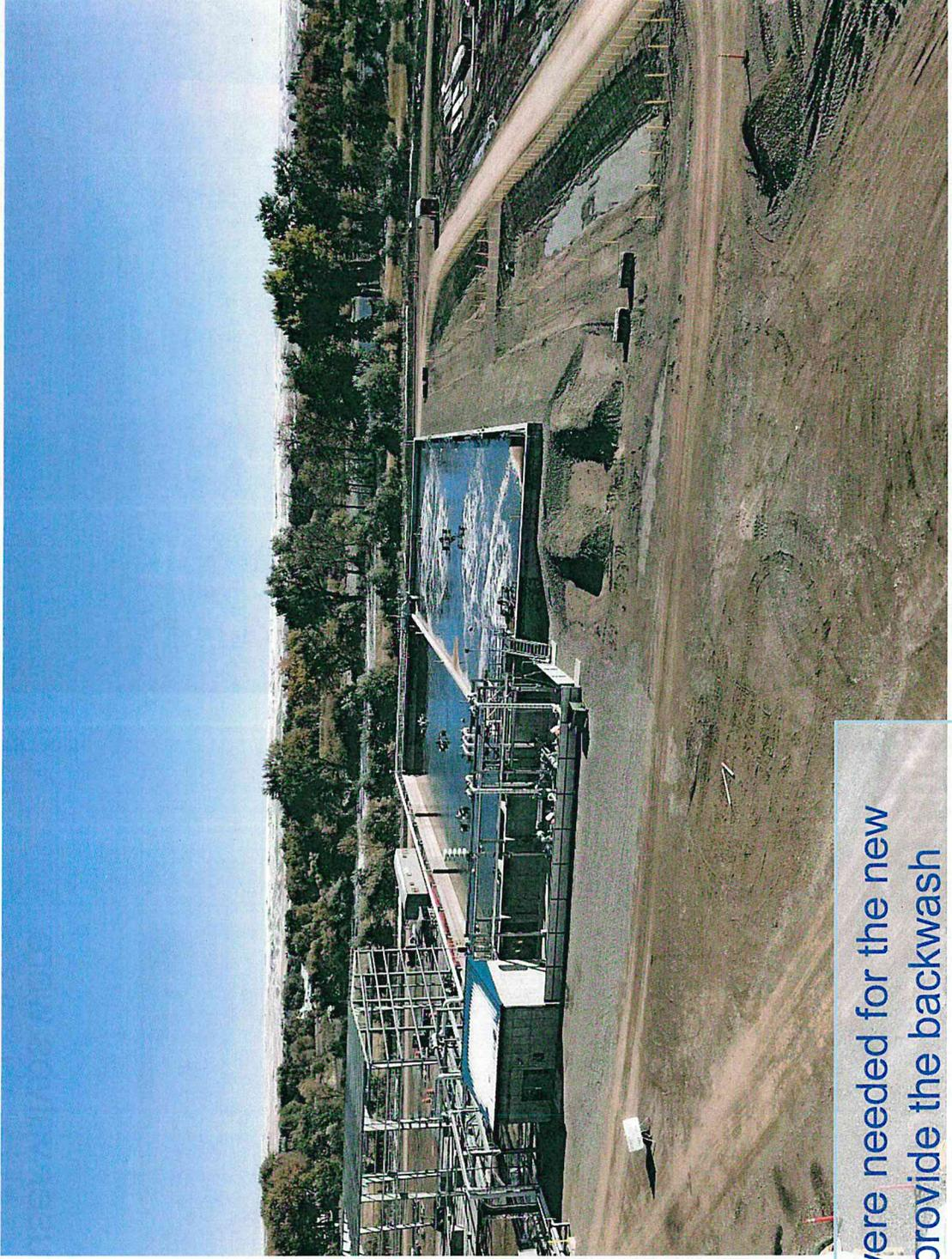
The new basins were needed for the new diffusers and will provide the backwash water for the new arsenic multimedia filters.
