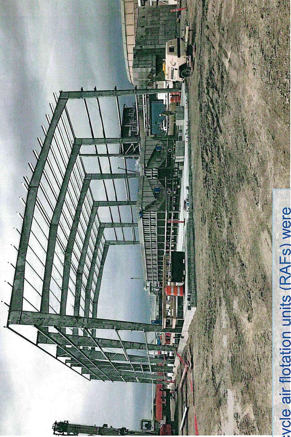
The two recycle air flotation units (RAFTs) were set before the building framework was installed.
