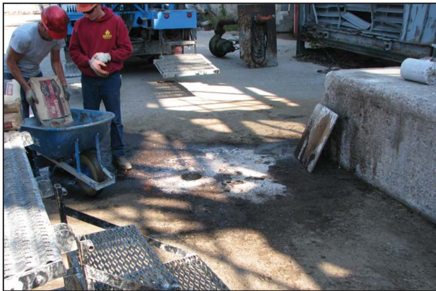
Completion of boring BB003 (Glue/resin wastewater tank).
