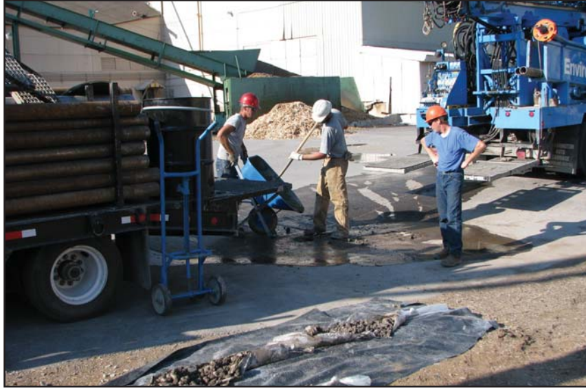
Completion of boring BB005 (Plywood Mill SE-side dry wells - North).
