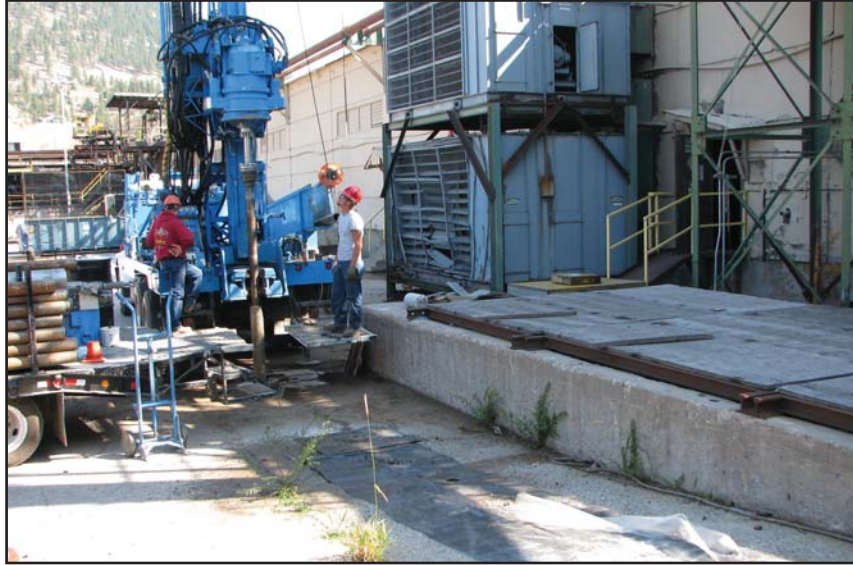
Advancement of boring BB003 (Glue/resin wastewater tank).
