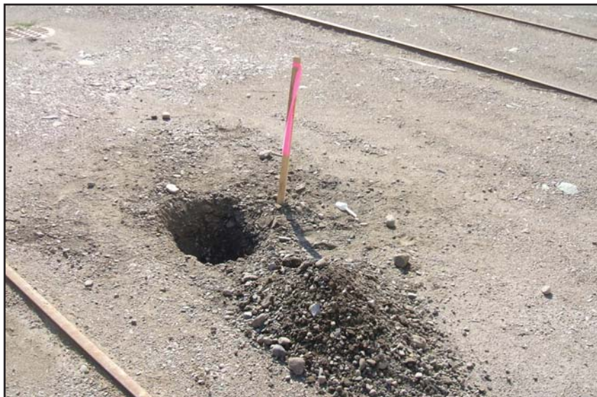
Advancement of hand auger HB001.
