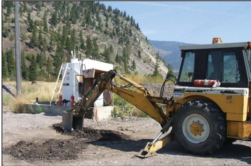
Advancement of test pit TB012 (East Log Yard).
