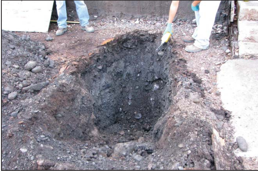
Petroleum-impacted soil observed in test pit at TB007 (Vat Area).
