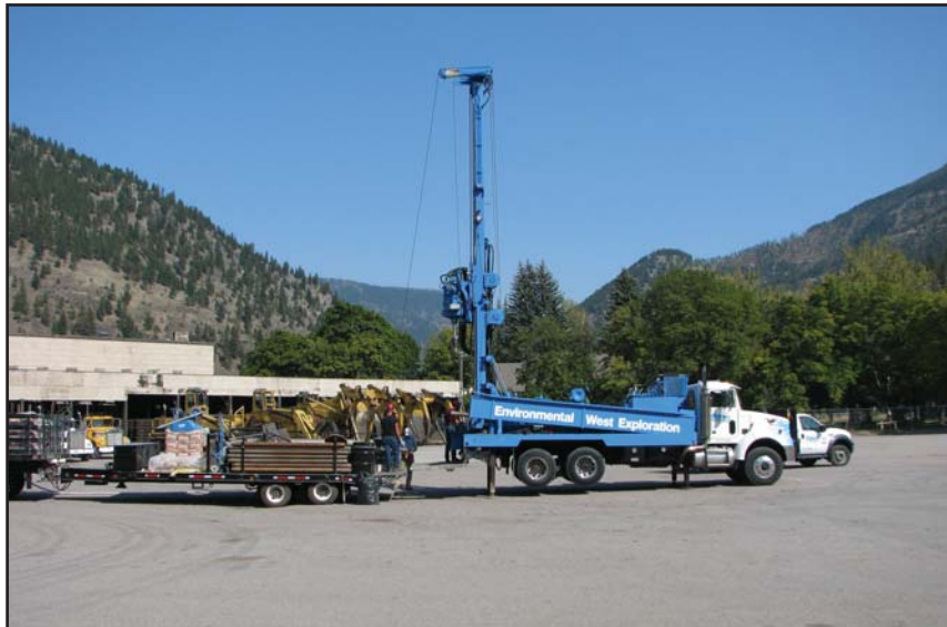
Advancement of boring BB012 (Dry Kiln Dry Wells).
